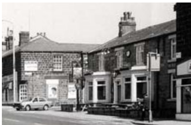
The New Inn, 1988 © Leeds Library & Information Service
